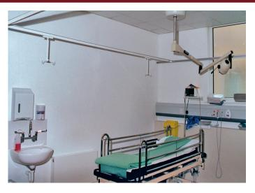
**Specification:** Movatrack IV400 Overhead intravenous track systems as supplied by Better Blind Company, 0800 169 3765. Extruded aluminium track with white powder-coated finish to be suspended (at 2.1m above floor level or as specified) in accordance with manufacturers instructions. 2-point carriers to be suspended from track on nylon runners. Layout as shown on accompanying drawings.
