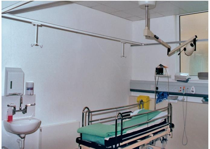
**Specification:** Movatrack IV400 Overhead intravenous track systems as supplied by Better Blind Company, 0800 169 3765. Extruded aluminium track with white powder-coated finish to be suspended (at 2.1m above floor level or as specified) in accordance with manufacturers instructions. 2-point carriers to be suspended from track on nylon runners. Layout as shown on accompanying drawings.
